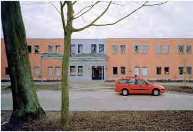
Teleportal clinic in Stolzenau Level access drive
